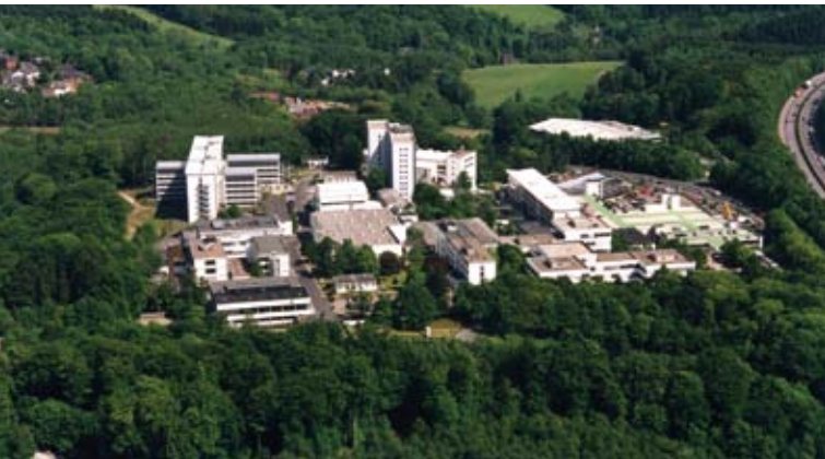
Technologiepark in Bergisch Gladbach.
